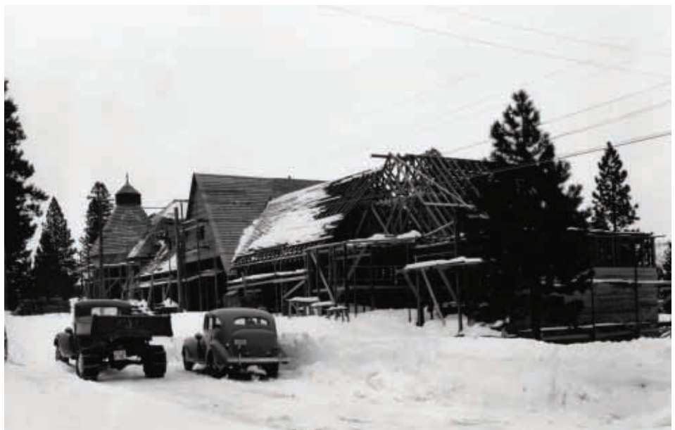
Ta-Neva-Ho under construction
